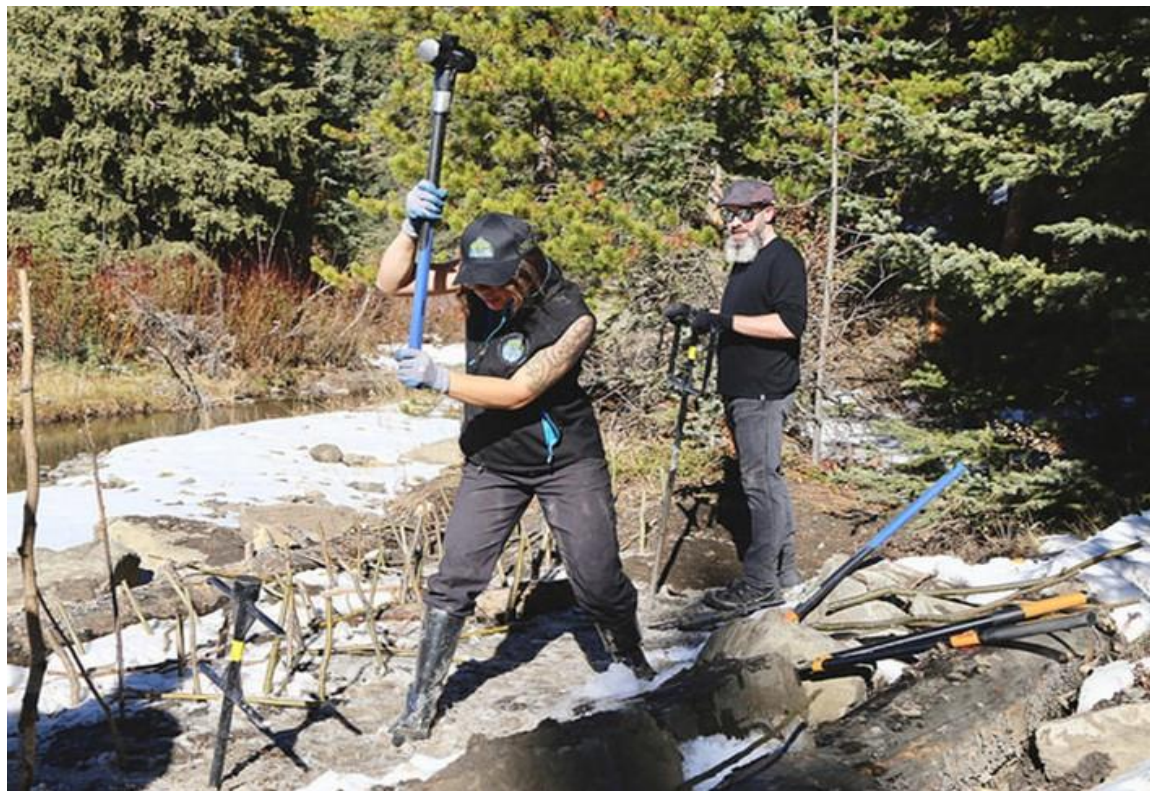
Staking willows to restore streambanks and reduce erosion at Pasque Creek.
